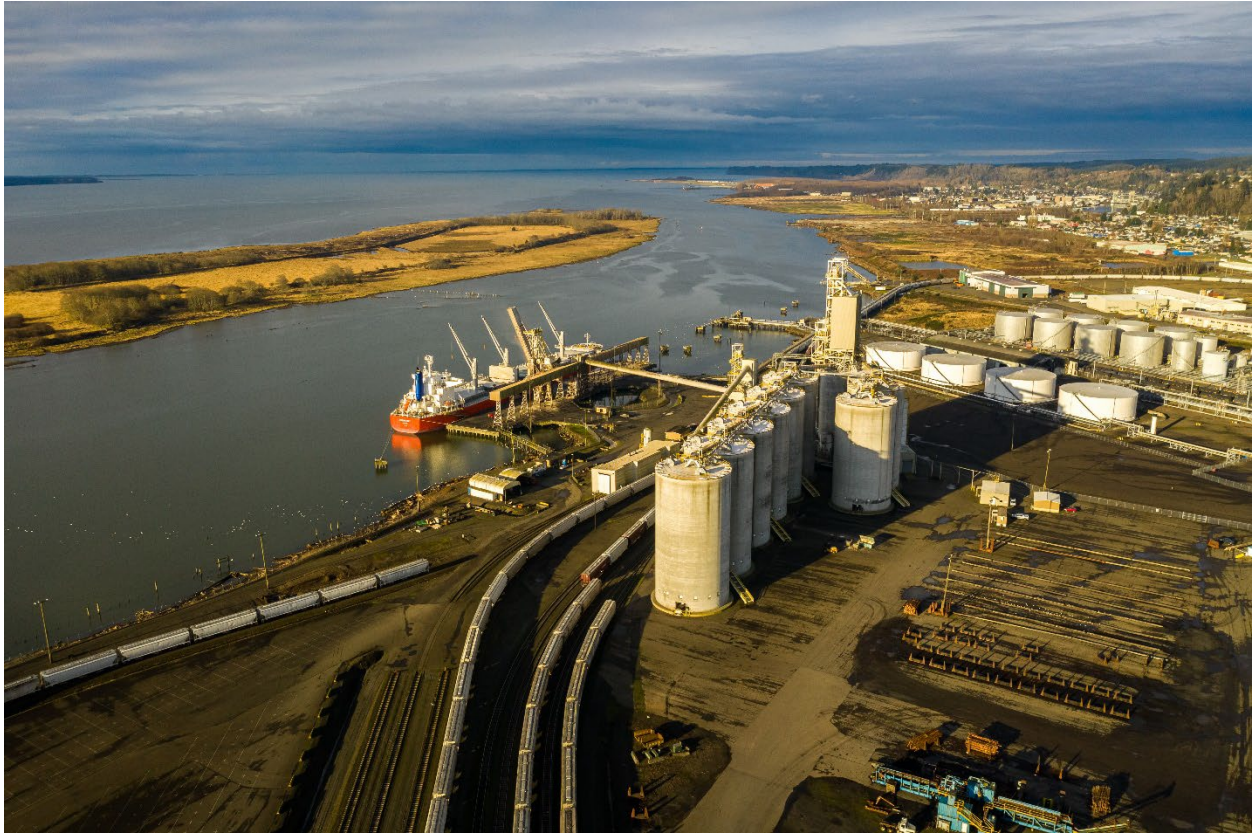
AGP announced plans for a new soybean meal processing plant in Nebraska on Friday. The Port of Grays Harbor stands ready to support AGP's export capabilities and expansion in Grays Harbor.
