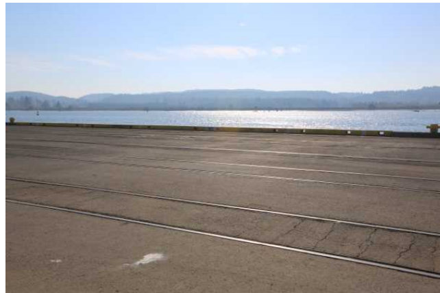
Dock, Looking Southeast
