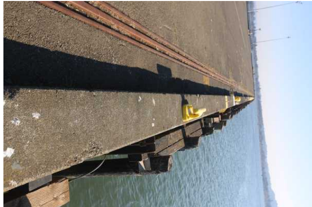
Detail of Curb and Bumpers at south edge.
