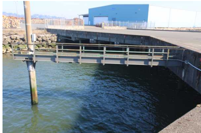
Detail of Steel Catwalk
