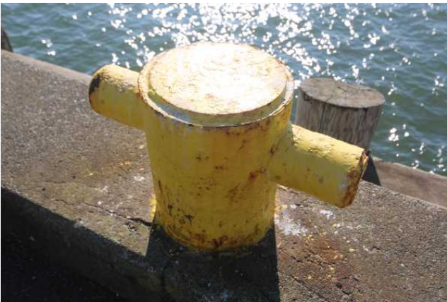
Detail of Mooring Ballard
