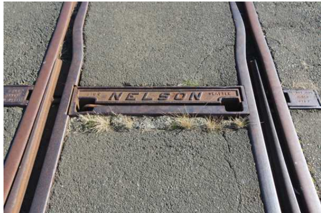
Detail of steel work at rail tracks.
