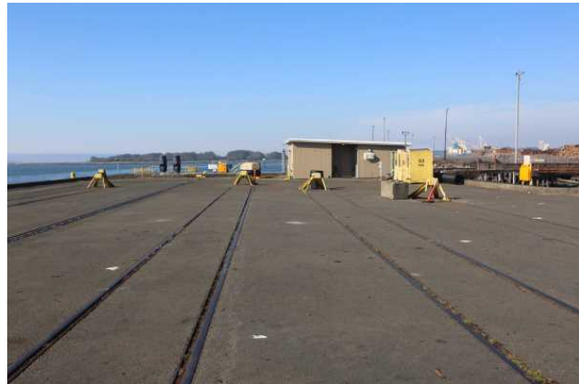
Dock, Western Section, Looking West
