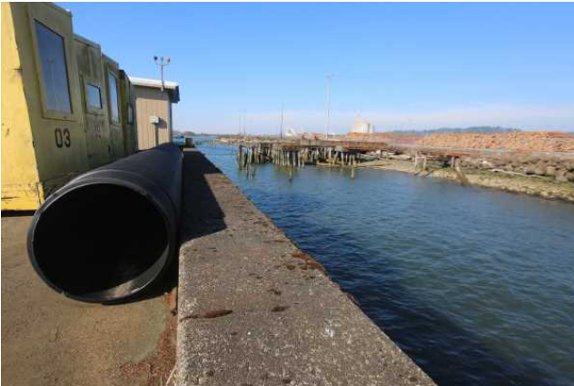
View of Dock's North Edge, Looking West
